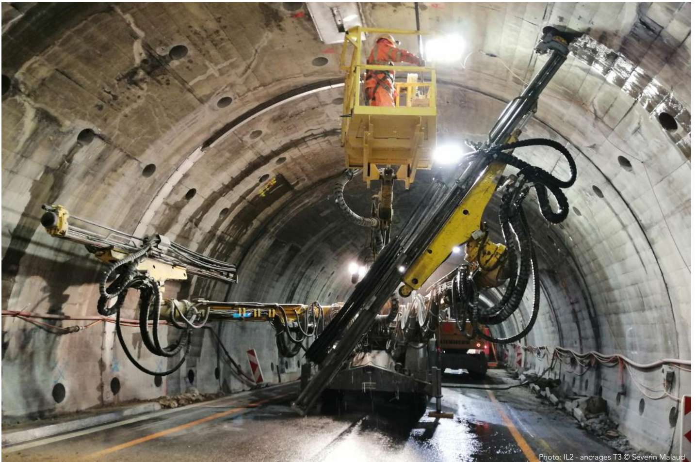
Photo: IL2 - ancrages T3 © Severin Malaud
